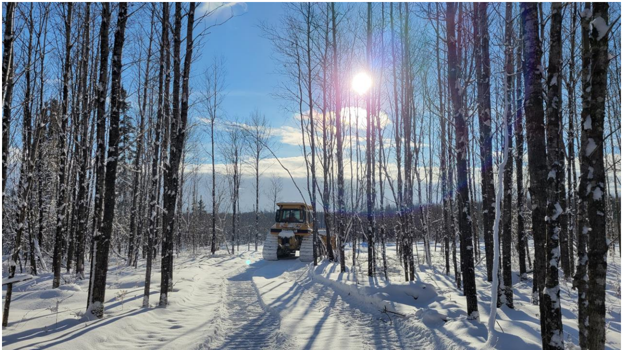
Photo 2: Dozer prepared access tracks and drill pads - Completed in March 2023
